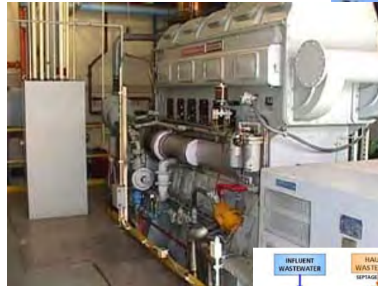
Back River WWTP AD/CHP (Three 1MW Gensets)
