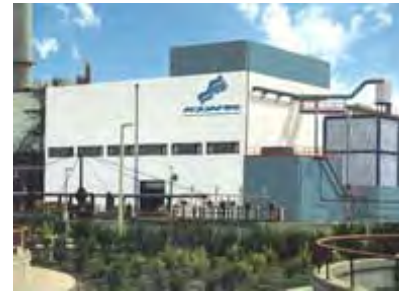
Keppel Seghers drying & combustion facility in Brugge, Belgium
