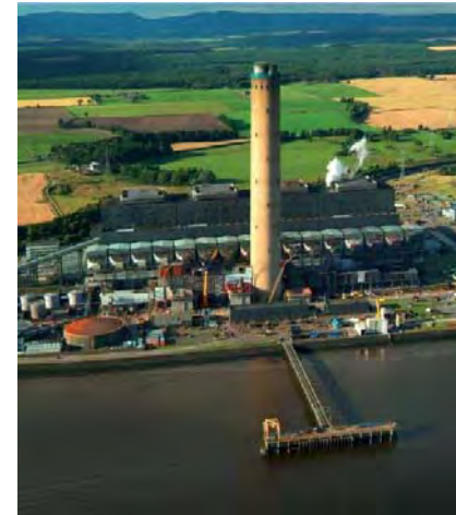
Scottish Power's Longannet Power Station
