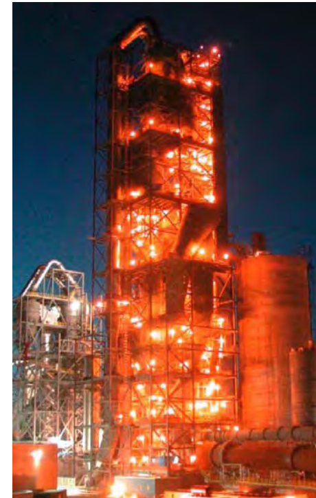
Lehigh Cement Plant at Union Bridge
